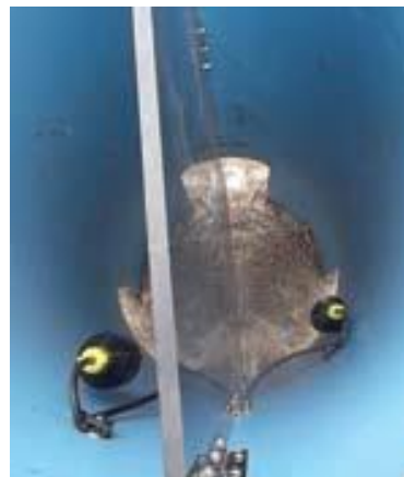
The blue cylindrical structure in the foreground holds the float switches and one gate valve. The Controller is visible in the background.
