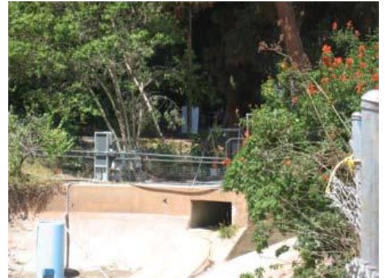
The blue cylindrical structure in the foreground holds the float switches and one gate valve. The Controller is visible in the background.
